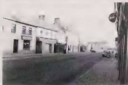
The view from the top of the hill towards the barricades (at Whelan's shop / Black Kettle).
