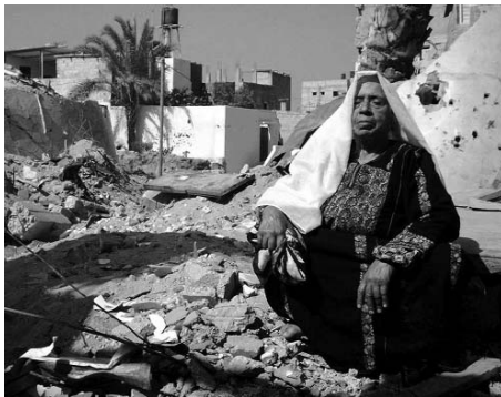
• A woman sits in the ruins of her demolished house in Gaza. The situation there is critical and aid is still being restricted by Israel (see left).
