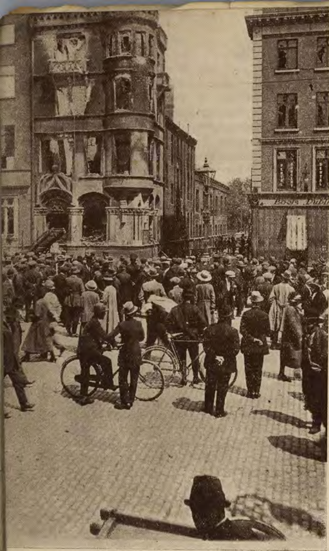
Dangerous Buildings being demolished
