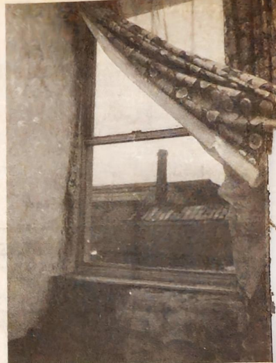
● Below the window ledge shown here is the black area of mildew which has appeared in many of the flats.
