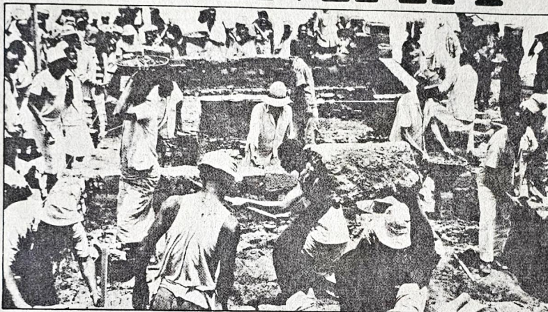
Communal building of new houses in an Ujamaa village
