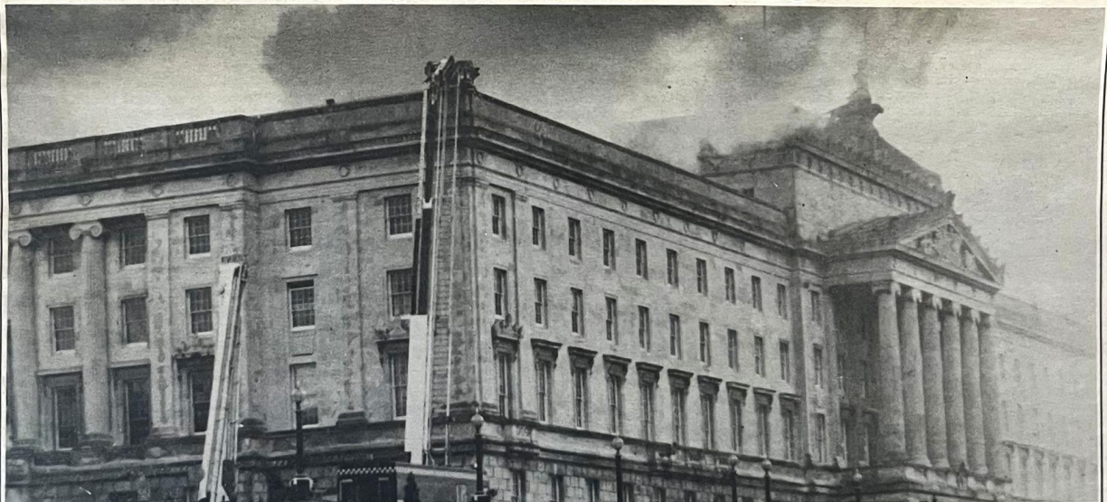
● Fire swept through the west wing of the Stormont parliament building outside Belfast on the morning of 2 January. Mystery still surrounds the cause of the blaze which completely gutted the debating chamber where the sectarian Six-County parliament sat until it was prorogued in March 1972. Nationalists have always regarded the building as a symbol of unionist and British misrule. DUP leader Ian Paisley claimed the fire was started deliberately, but British government and RUC spokespersons said the cause was as yet unknown
