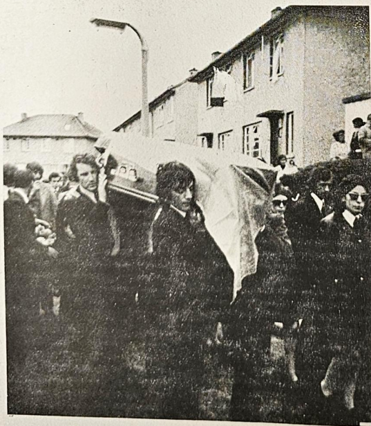
Remains being carried from home.
