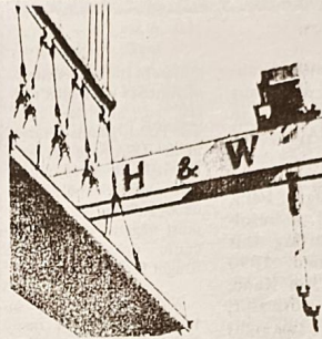
Throughout this 39-page, A4 size report the figures are well-presented and easy to read and the accompanying text is punchy and succinct. At £1.50 it is accessible to all.
