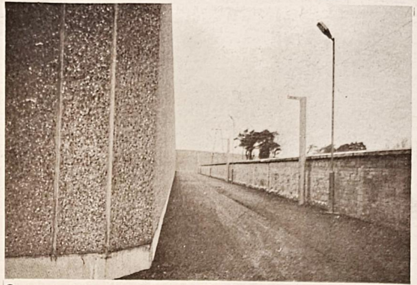
● Perimeter Wall of Wheatfield Prison, Clondalkin.
