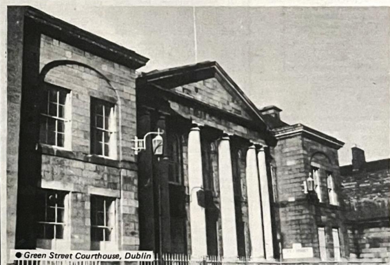
● Green Street Courthouse, Dublin
