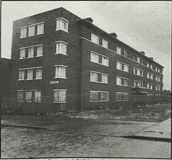
Part of the Sheriff Street Flats complex in Dublin's inner city
