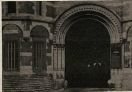
● The imposing entrance of Strangeways Prison, Manchester, from where six republican prisoners escaped in 1919
