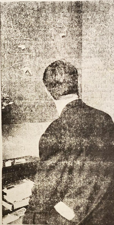
● Bullet-holes in sitting room wall at Ladbrook Drive, Ardoyne, Belfast.
